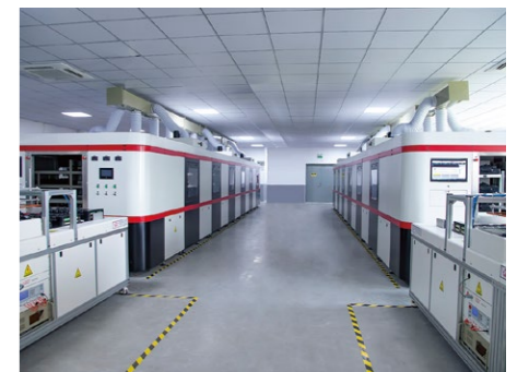
Automatic Aging Test Workshop
